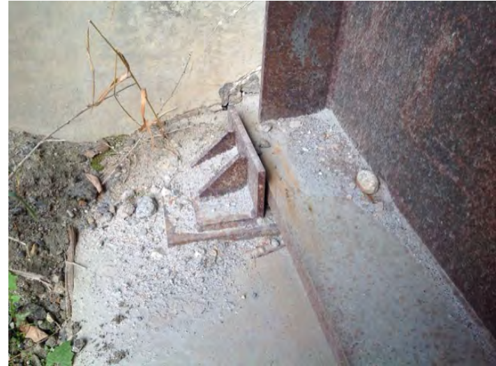
right bank girder bearing keepers - typical
