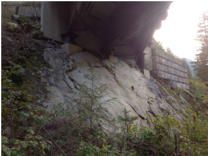
Left Bank Abutment when facing downstream
