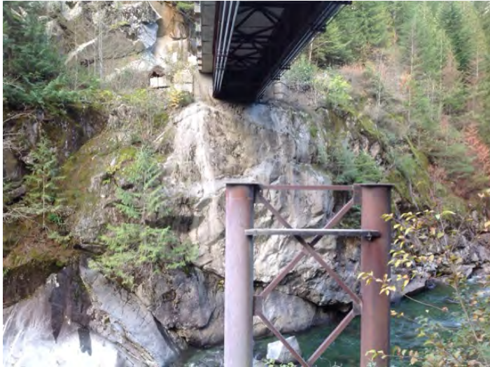
Right Bank Abutment when facing downstream
