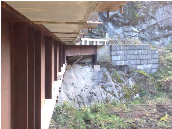
downstream left bank girder flare
