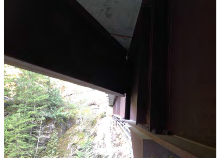
left bank girder flare
