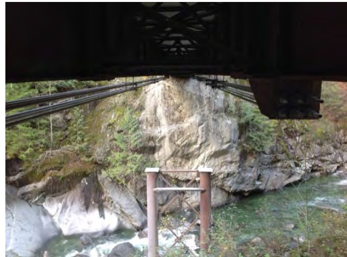
Right Bank Abutment when facing downstream
