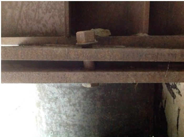
upstream left bank bearing bolt
